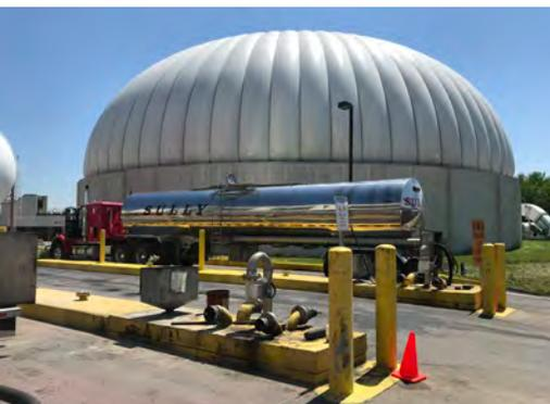
“Net Zero.” For the Greater Lawrence Sanitation District in Andover, MA CDM Smith expanded the existing digestion facility and added a combined heat and power system to enable acceptance of food waste into the digesters to increase gas production. Again, not only did the District receive revenue from tipping fees but also received the benefit
